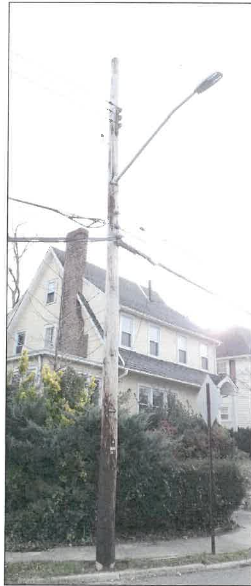
1 EXISTING POLE PHOTO SCALE: NTS
